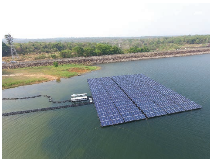
Fig. 2.11 : Demonstration of 249.6 kW p FPV at Sirindhorn Dam, Ubonratchathani Province
